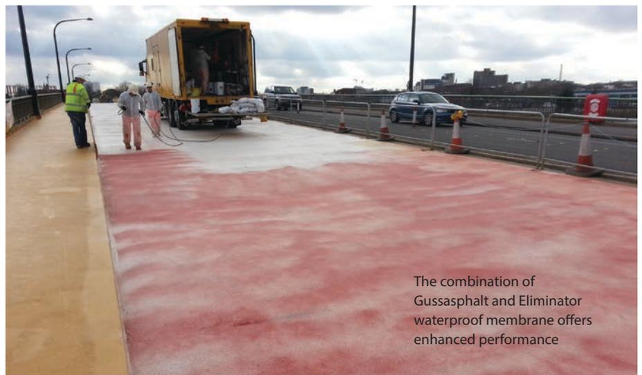
The combination of Gussasphalt and Eliminator waterproof membrane offers enhanced performance
